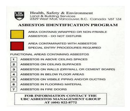
Sample asbestos identification door sticker indicating floor, above ceiling and wall materials contain asbestos:
